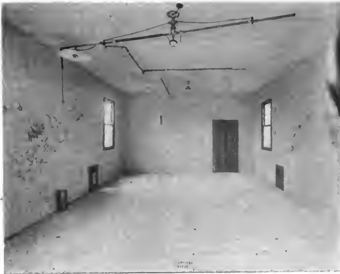
Interior of Garage Part of Hollow Tile Building
